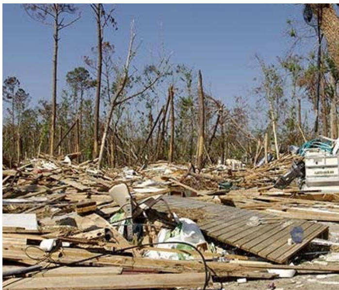
A Mississippi home leveled by Hurricane Katrina. While many houses have been rebuilt, much remains to be done.
